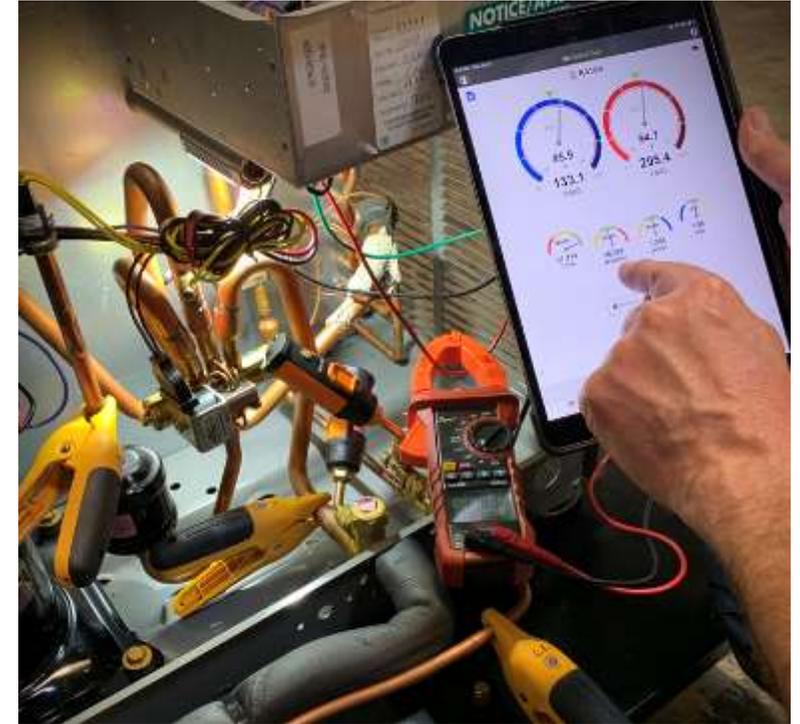
**Solution:** Smart diagnostic tools help ensure heat pumps are installed properly, resulting in realized energy-efficiency and reduced energy waste.
