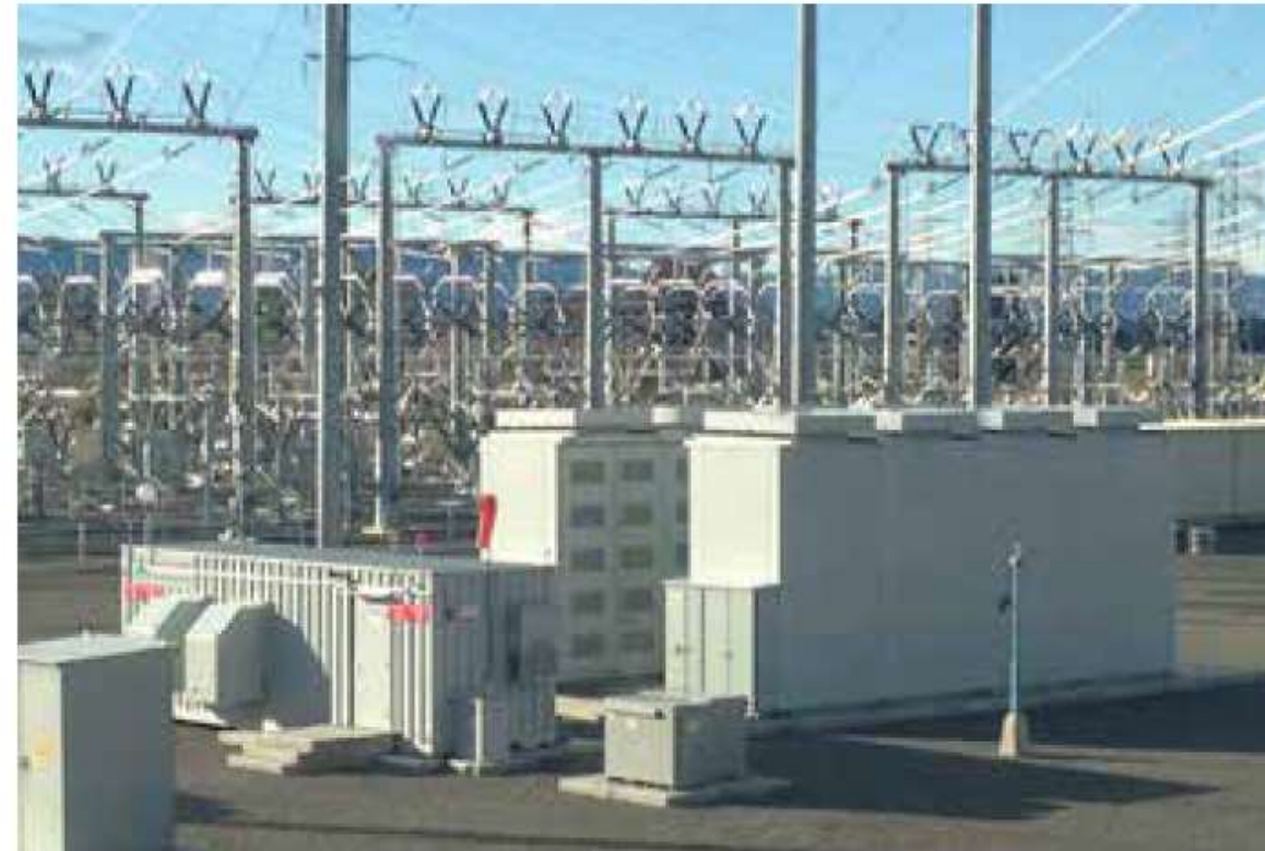
Photo Credit: Pacific Gas and Electric Company
