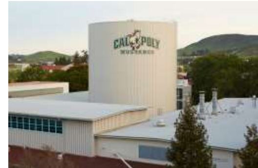
Cal Poly's Thermal Energy Storage Tank Source: Cal Poly
